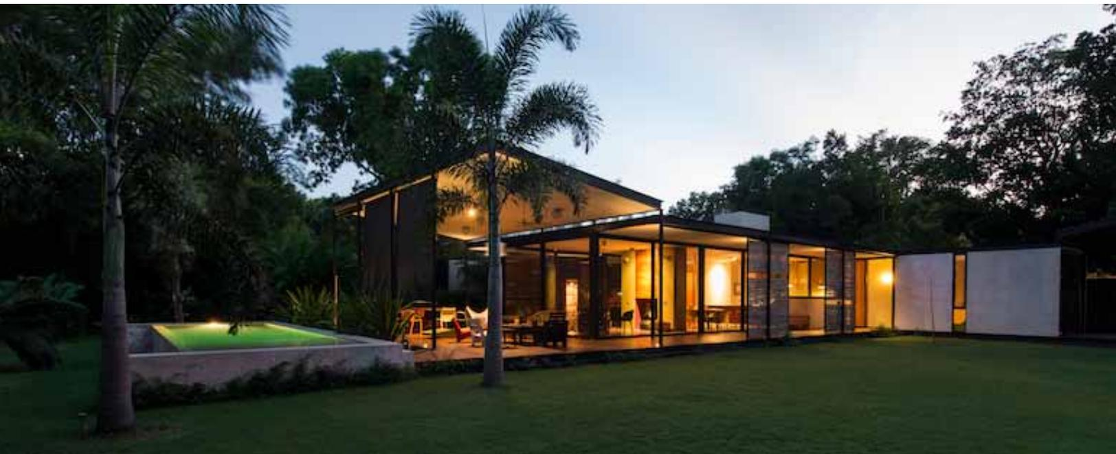
The architecture is defined in the congruence between the rational logic of use of materials and the plastic tectonics that the construction system revealed to us as design opportunities. From this the spaces are designed in relation to different layers of protection: ventilated floors, overhangs that are circulations and light-temperature transitions, sliding-pivoting metal panels with bamboo from the region.
