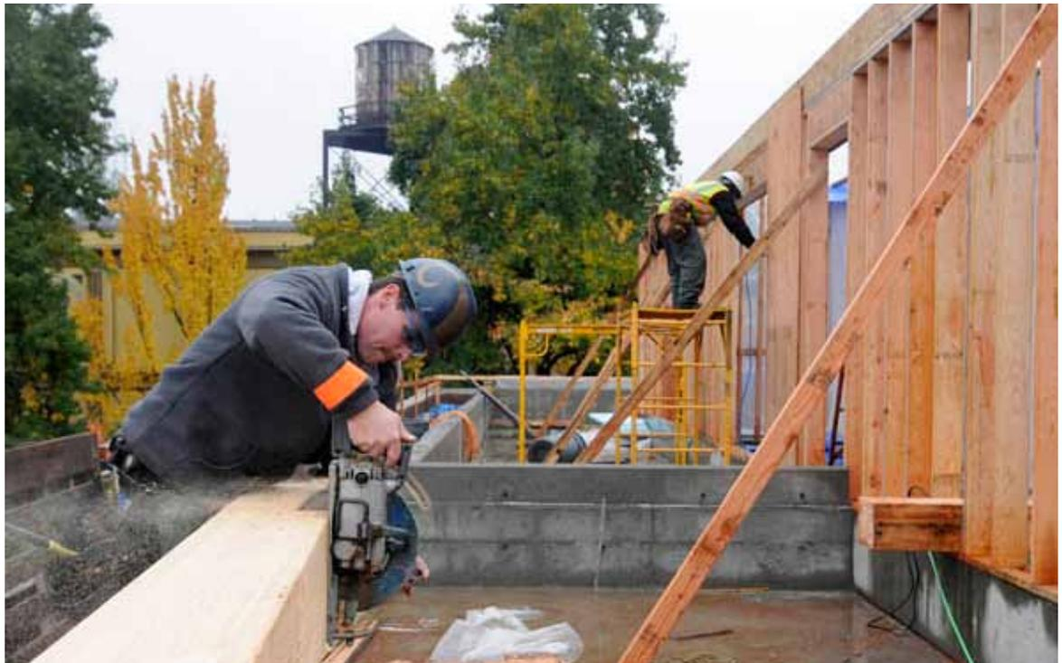
*Sam Sibold, an apprentice carpenter with Time Frame Inc., nails a rim joist on the top floor of the future OCOM campus in Old Town.*
