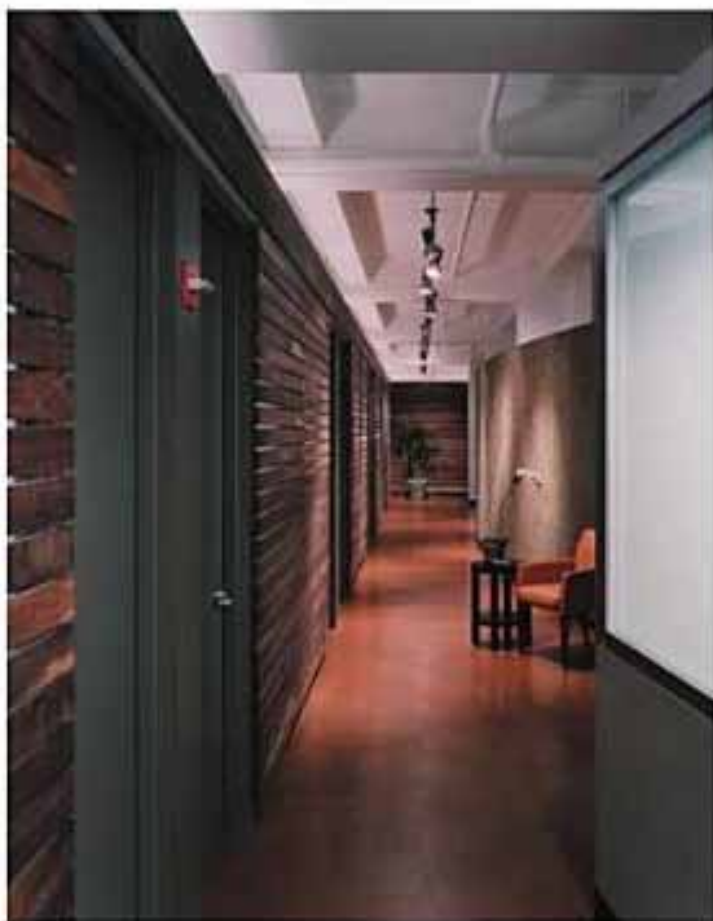
Wood reclaimed from abandoned buildings finds new life in the wood slat wall of this corridor. It is finished with a natural oil that is completely biodegradable and emits no VOCs. © Peter Mauss/Esto
